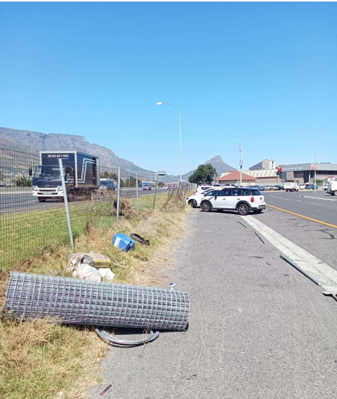
Fence repaired after N1 accident
