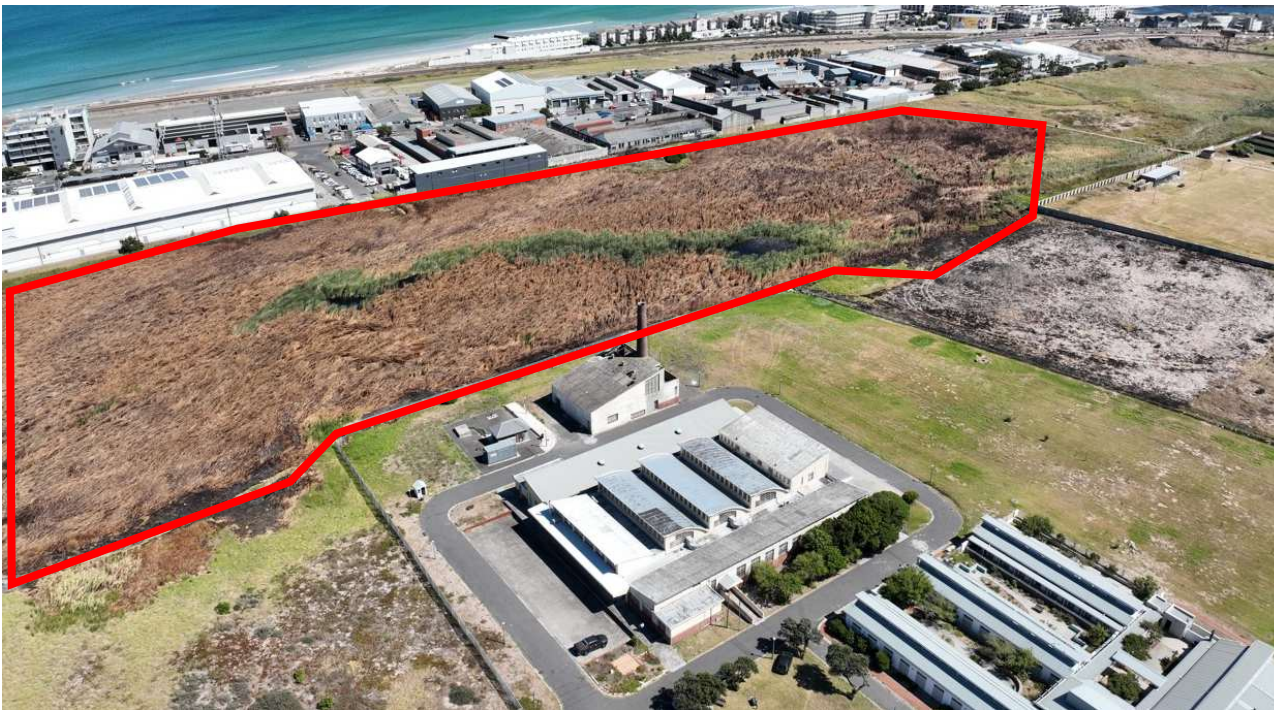
FIRE AFFECTED AREA IN ZOARVLEI MARKED IN RED
